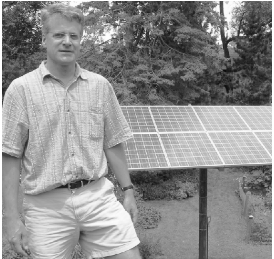
Niels Wolter stands above a 1.264 kw, dual axis, grid-connection solar array in the backyard of his Madison home. A second solar installation on the house's front roof provides hot water.
